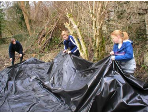
2. The special butyl liner is carefully manoeuvred into place.
