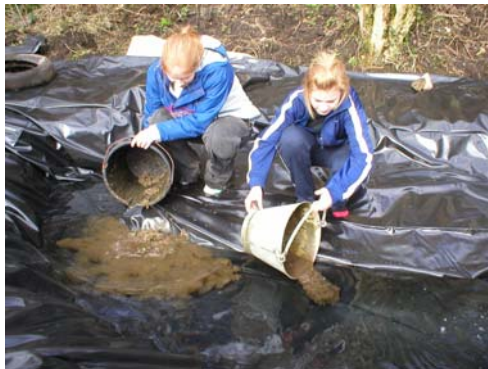
4. Water and silt from a neighbouring pond is added to give a helping hand.
