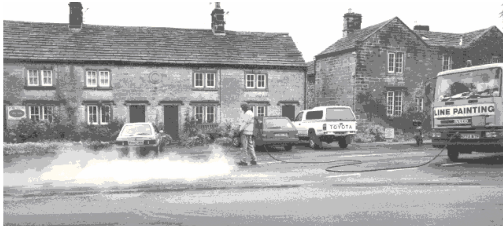
Middleton Village Square with the unnecessary work being undone
