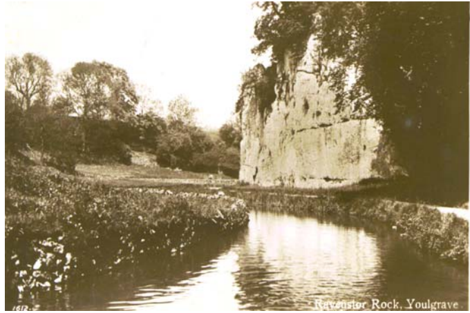
Raenstor Rock, Alport. The top portion you can see here had to be blasted away as it had become dangerous to users of the coach road.
